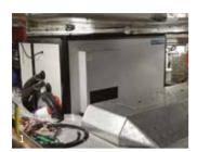
In order to meet our structure-borne noise requirements we designed a new base frame concept (1). Through FEA and specific mount selection (both single and double) an optimal result can be achieved.
